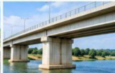
Bridge Construction Safe and durable structures.
