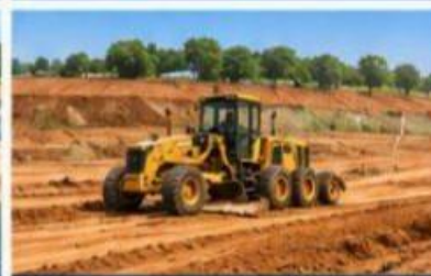
Site Development From earthworks to complete infrastructure.
